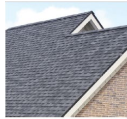
Asphalt shingle roof
